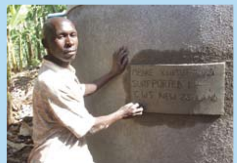
The finishing touches to a rainwater tank.
